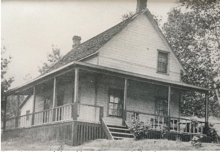
Francis Harvey's hand hewn square timber home. Later covered in wood siding by the new owners. Story and picture courtesy of Dorset Heritage Museum
